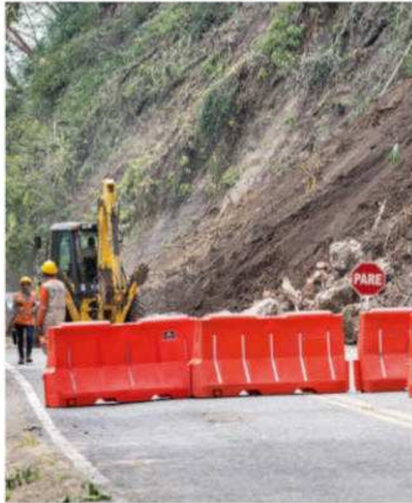
Removing road blocks
